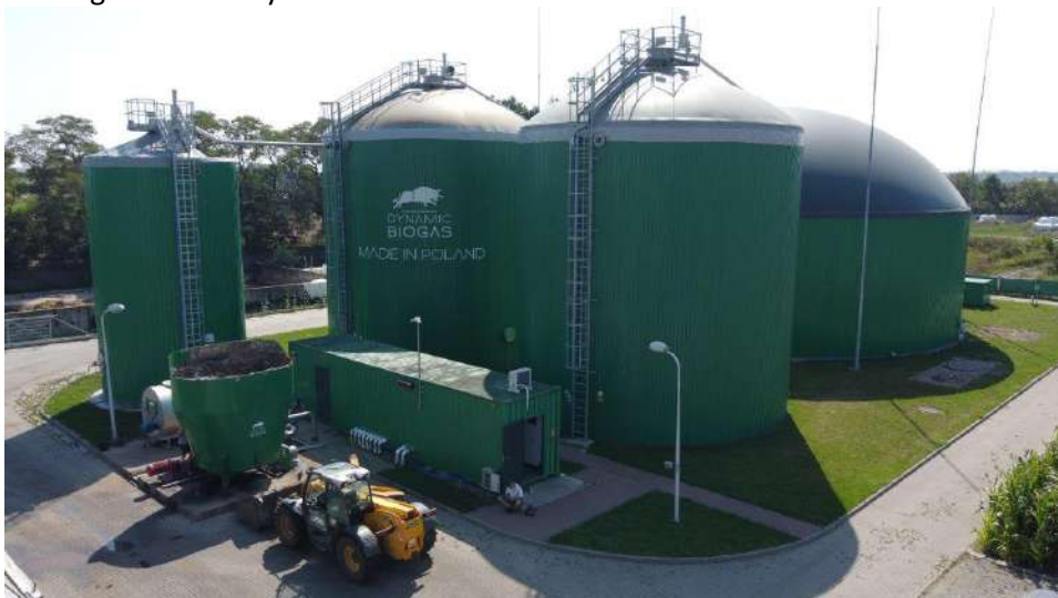
Figure 1. Biogas plant (499 kW of electric power) in the Przybroda experimental farm with dairy production related to Poznań University of Life Sciences
